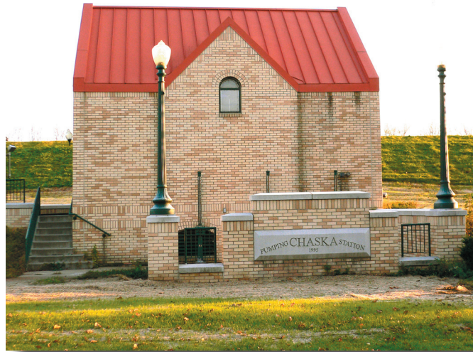
Pumping Station constructed in 1995
