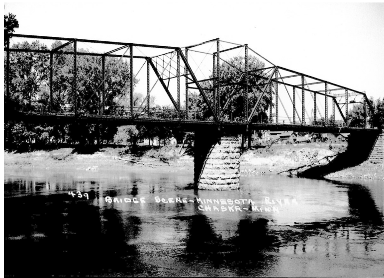
Historic truss bridge on Highway 41
