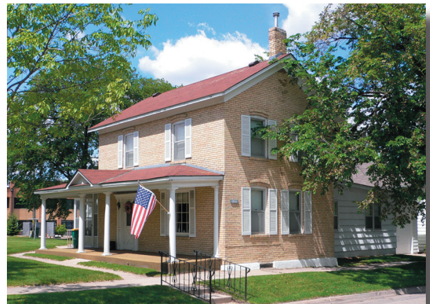
Colonial Revival details are found in the Chaska brick home at 415 Walnut Street
