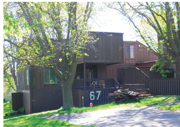
Notice the multi-angled shed roof and the vertical wood siding on this home in Jonathan's Neighborhood One
